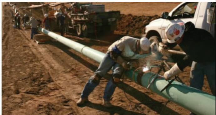
Installing New Natural Gas Pipelines (Image: Real Clear Energy)
