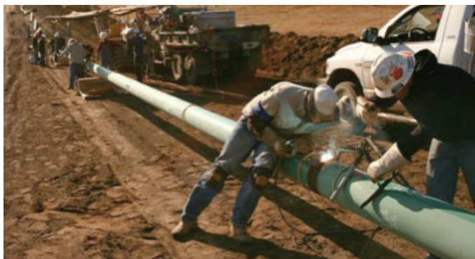
Installing New Natural Gas Pipelines (Image: Real Clear Energy)
